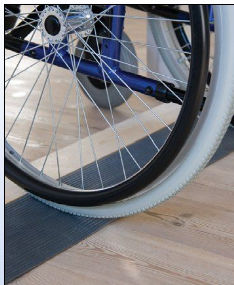
LX1a. Rubber ramp in use
